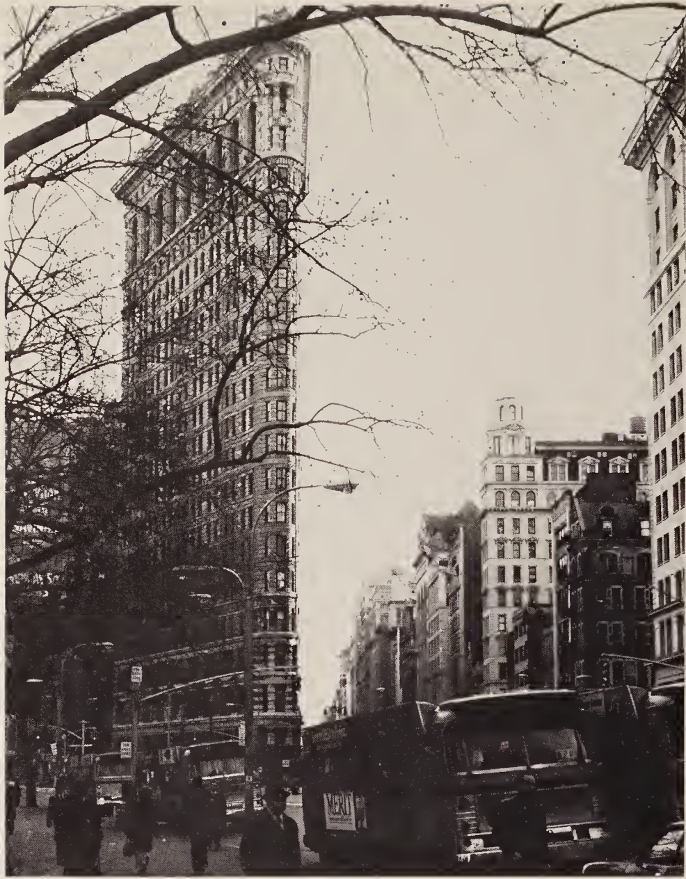
Photo/souvenir The Iron Building, New York, March 1976.
